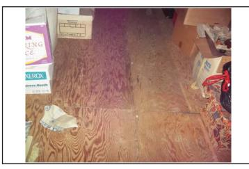
Floor boards cover 40% of your attic. Add dense pack cellulose to fill cavity under the floor boards.
