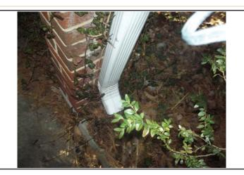
Divert downspouts away from the house (at least 5 feet) to ensure proper drainage and to prevent moisture and structural issues in the home.
