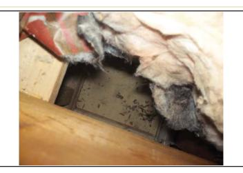
Seal this framing void in the attic.
