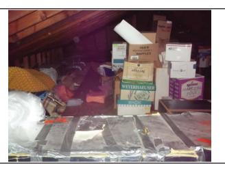
The existing attic insulation is only 6". Add an additional 12" of insulation to the attic to bring level to R-49. Obstructions will need to be removed.
