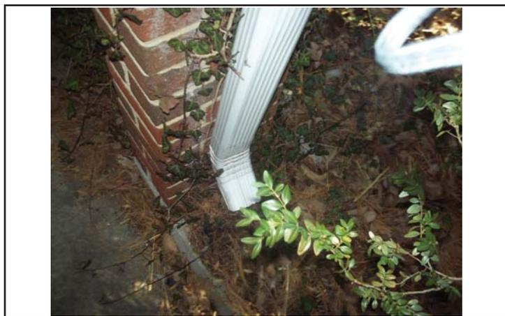
Divert downspouts away from the house (at least 5 feet) to ensure proper drainage and to prevent moisture and structural issues in the home.
