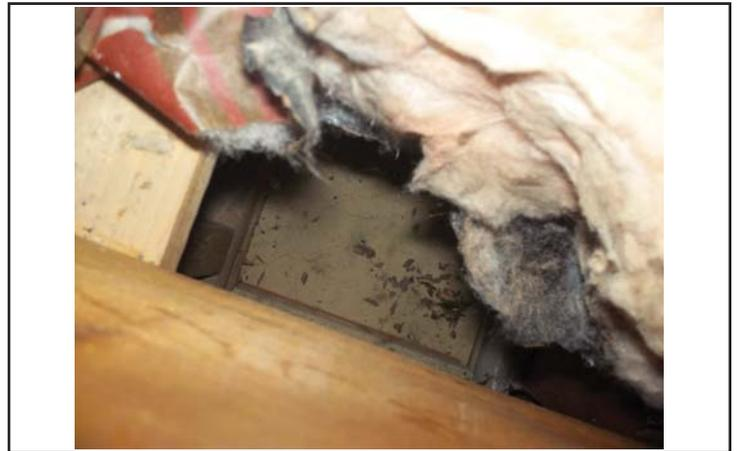
Seal this framing void in the attic.
