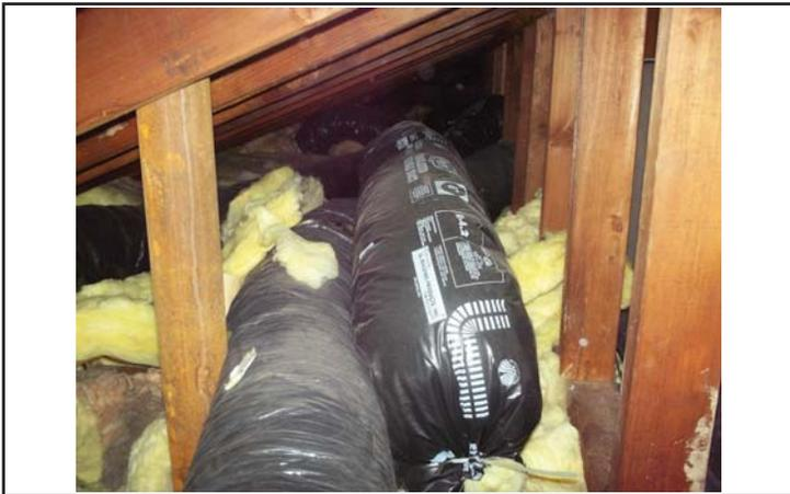
Bury all accessible duct work in cellulose when adding insulation.
