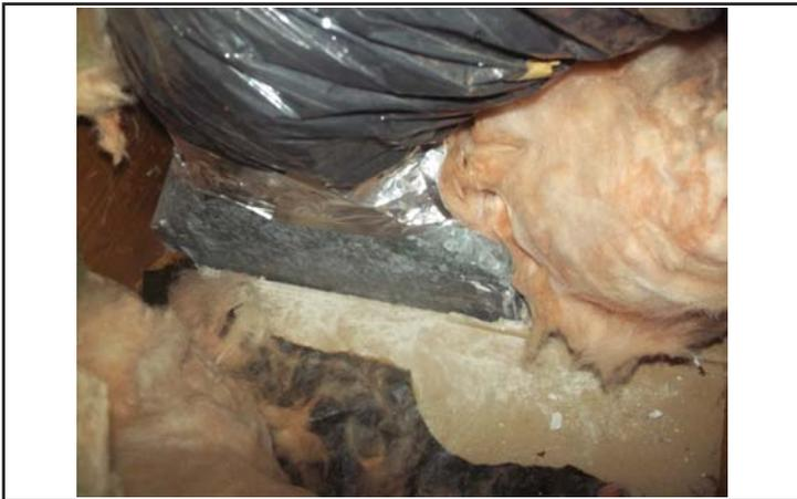
Seal the duct penetrations in the attic.
