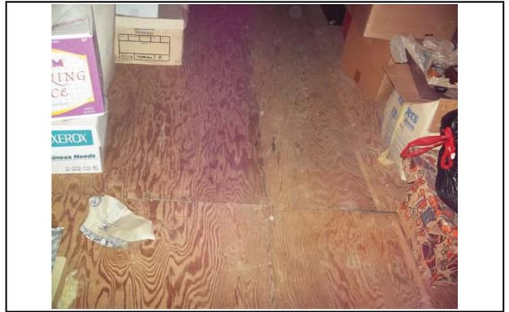
Floor boards cover 40% of your attic. Add dense pack cellulose to fill cavity under the floor boards.
