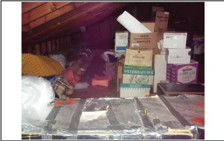
The existing attic insulation is only 6". Add an additional 12" of insulation to the attic to bring level to R-49. Obstructions will need to be removed.
